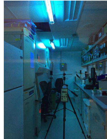
Ceiling UV light used for air and surface disinfection
